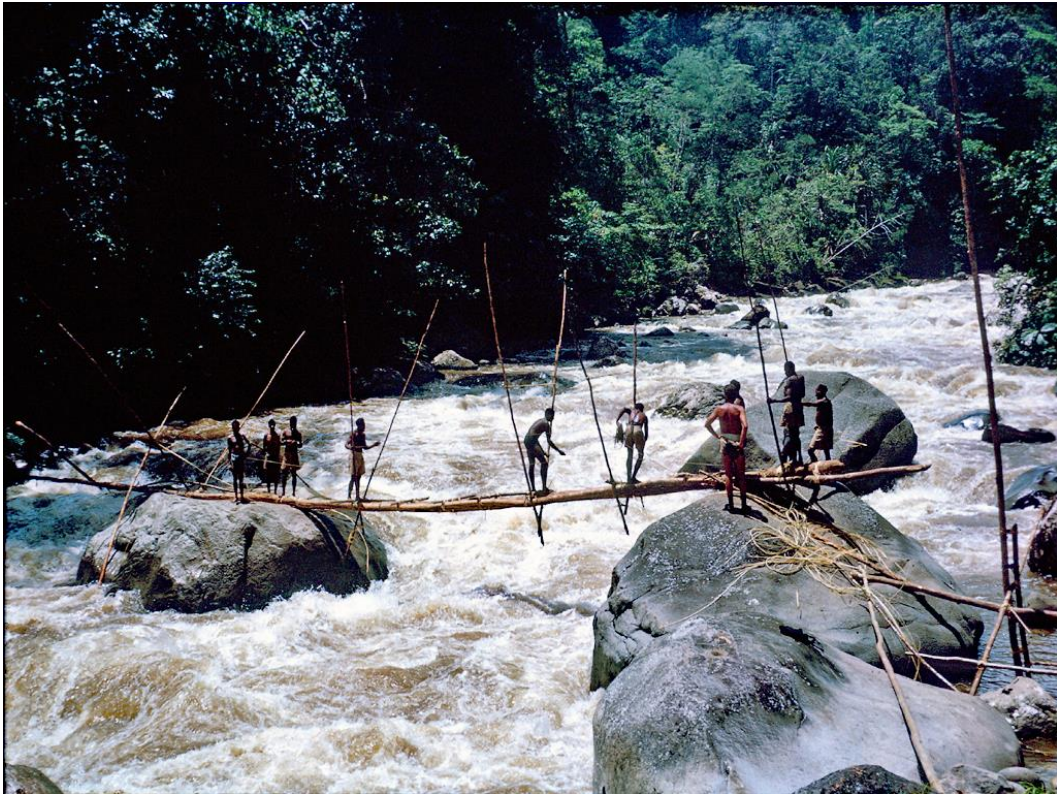
Bun River Bridge 2
