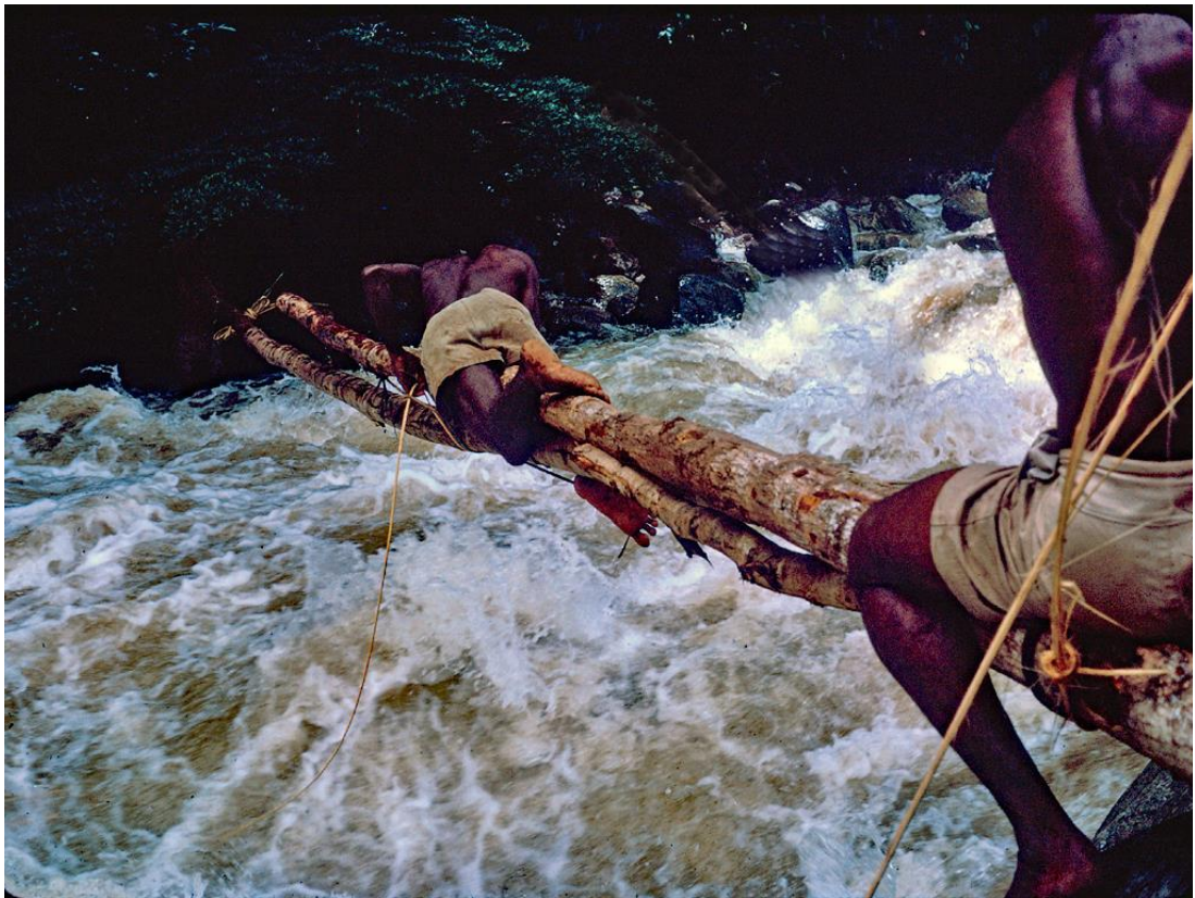
Bun `River Bridge (or part of)
