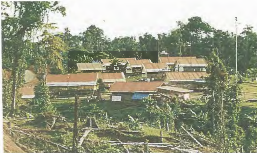
Above - Kumul camp on the bank of the Fly River at Drindmasuk. Bush timber frames, split palm floors, plastic sheeted walls and tarpaulin rooves.
