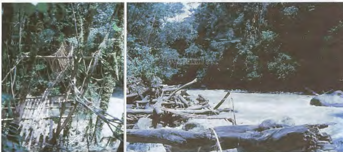
Above - Cane swinging bridge, built entirely from forest products in five hours
