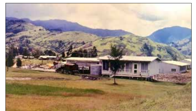
Sunken graders and tracked loader near Kerowagi (top); Rolled Mack 10-wheeler fuel tanker, Lower Daulo Pass (second); Road collapse caused by guria —dozers cutting a new alignment, Chuave (third); The house at Kundiawa with the works depot in the background (bottom).
