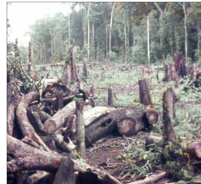
Cleared Usino-Dumpu road alignment, preceding earthworks
