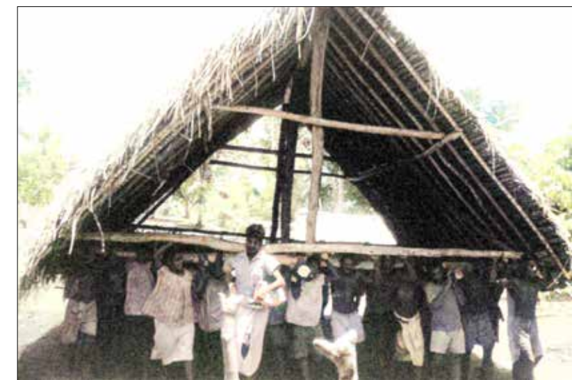
Moving the classroom roof to the new structure
