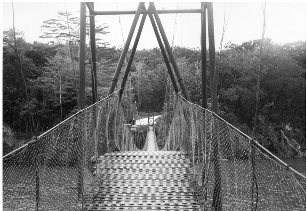
The bridge built from scrap metal across the Mape River
