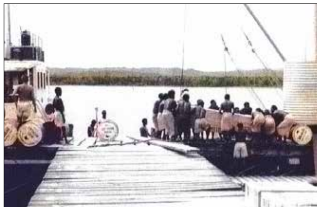
Kuku Kuku prisoners unloading cargo at Kerema for the new airstrip
